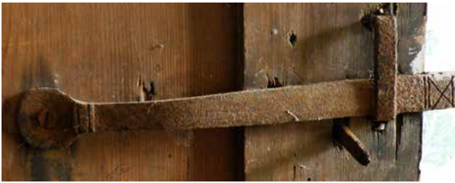
Figure 27. X-mark on the latch of a cellar door, c1720.
