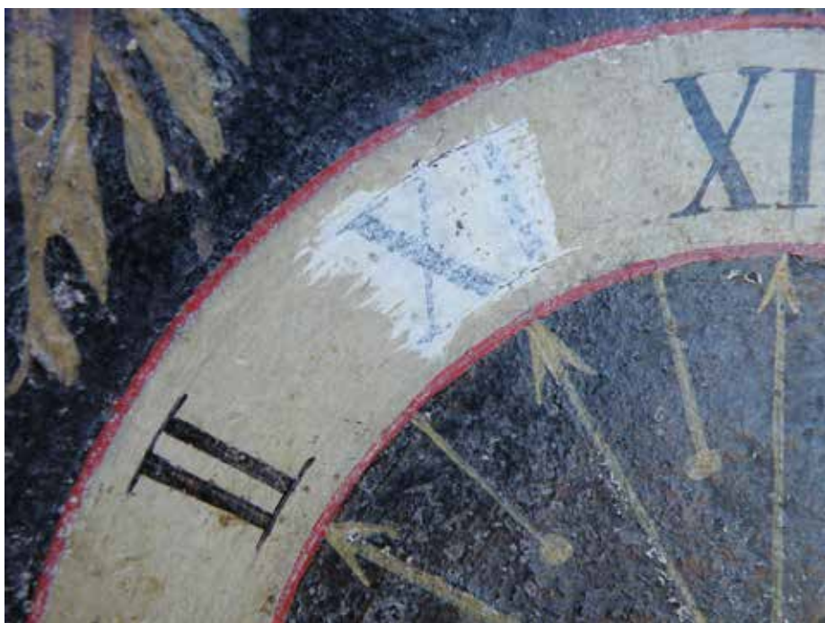
Figure 14. The original XI revealed beneath the later anti-lockwise hour numerals.
